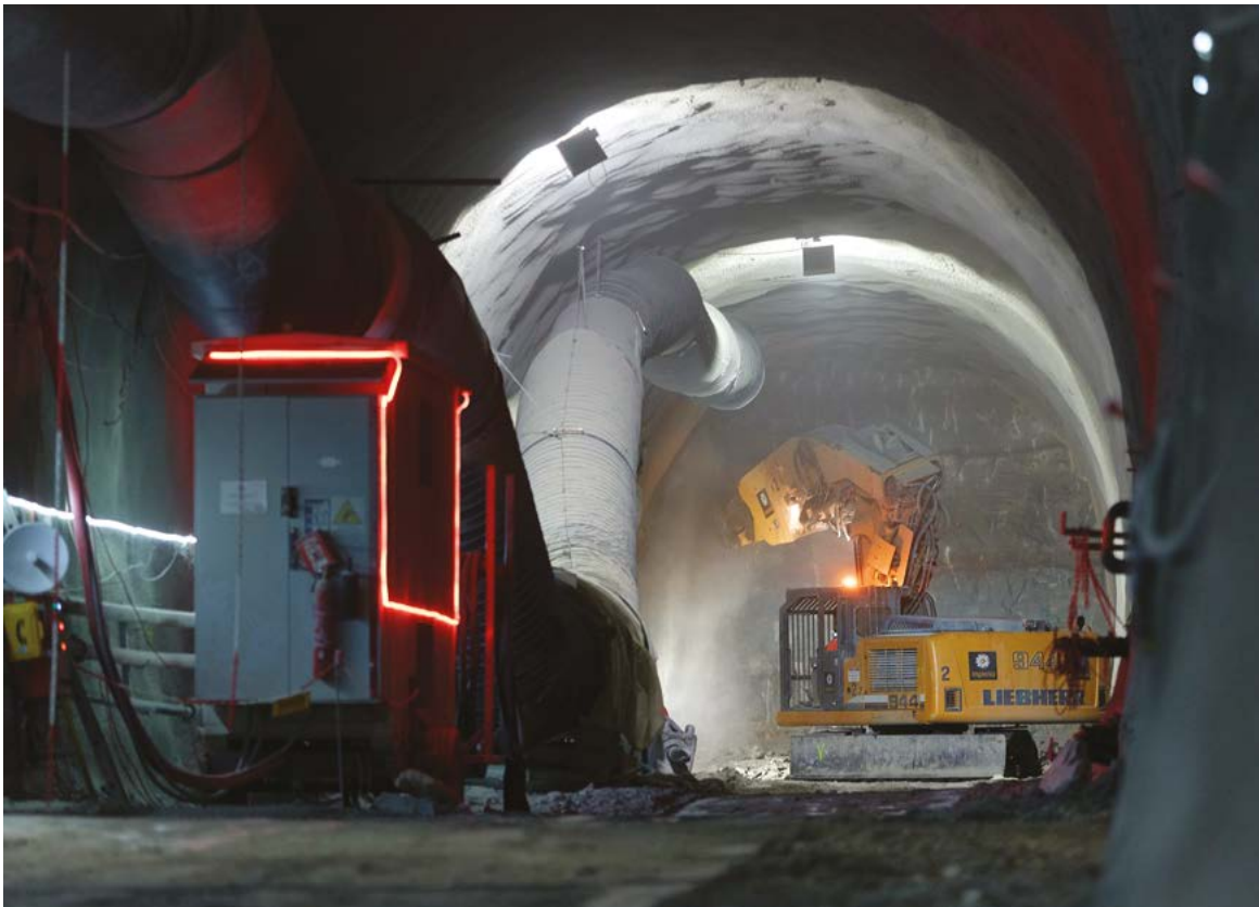
Excavation works for the High Luminosity LHC at CERN in 2023. Credit: CERN
